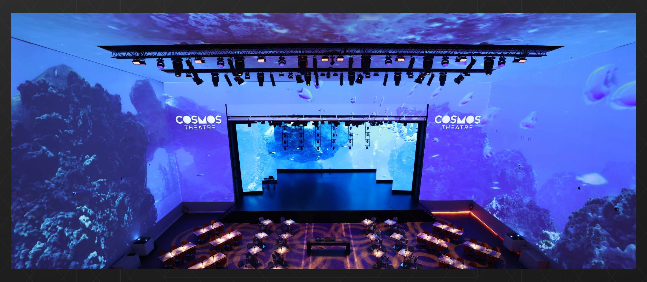
Cosmos Theatre possesses a 1200 square meter mapping area created using silver-colored acoustic fabric (PONGS) that maintains sound quality while keeping speakers out of sight and enhancing visual quality. The 270° mapping system, facilitated by 32 projectors, allows the space to transform into any desired arrangement.
